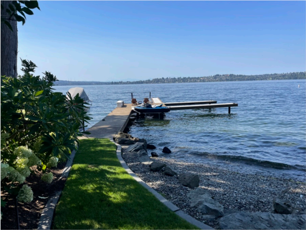
Photo 1 - Existing dock looking waterward.
