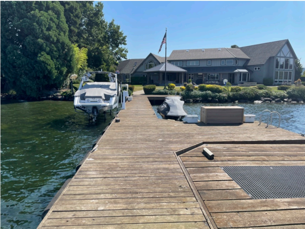
Photo 2 - Existing dock looking landward.
