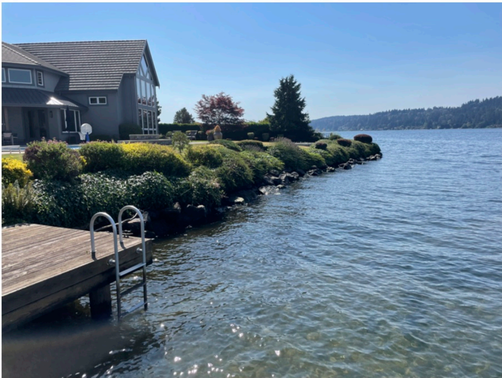
Photo 4 - Shoreline conditions south of the dock.
